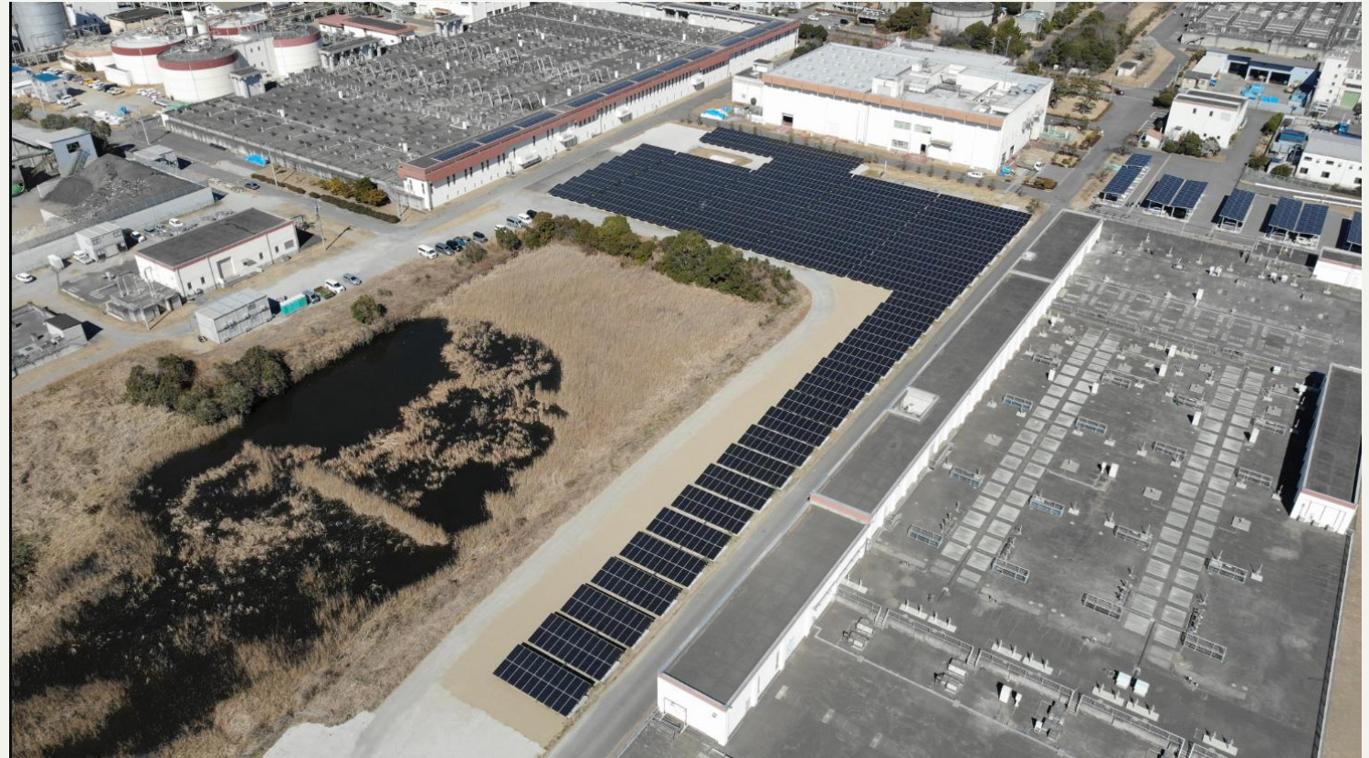
Solar power generation facility at the Chiba City Nanbu Sewage Treatment Plant
