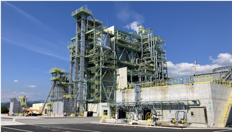
Hyuga Biomass Power Plant Start of operation: Oct. 16, 2024 Output capacity: 50 MW Orders: O&M, LTSA, etc.
